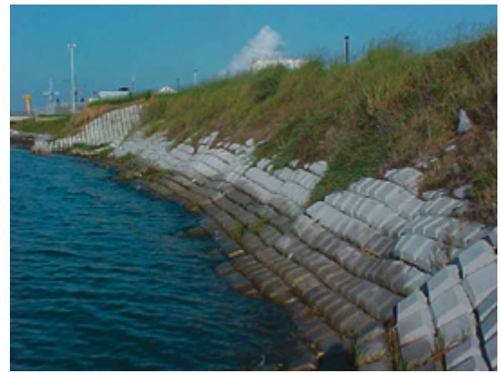
Photo: Koch Pipeline Company
