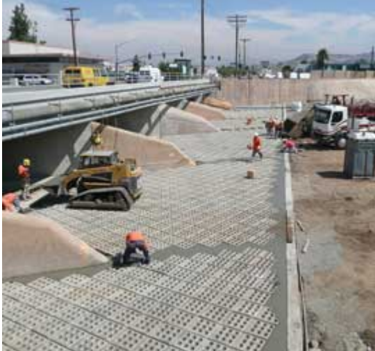
Photo: Soil Retention Articulated concrete blocks reinforce the channel bottom.
