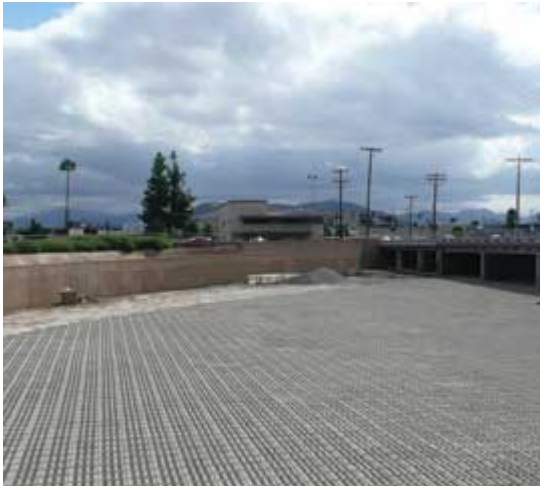
Photo: Soil Retention The newly restored Forester Creek channel can accommodate a 100-year flood.
