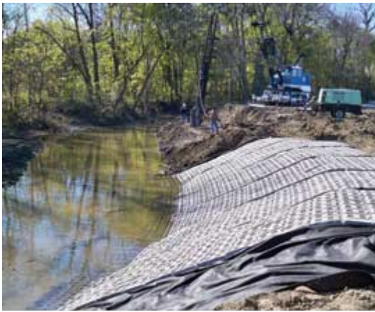
Photo: Charles E. Leser, Madison County The mats that were used had about a 20% open area through which vegetation could grow.
