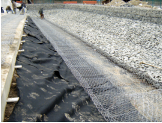
Photos: Maccaferri Gabions can be used to form natural drainage systems, minimizing the buildup of hydrostatic pressure on streambanks.
