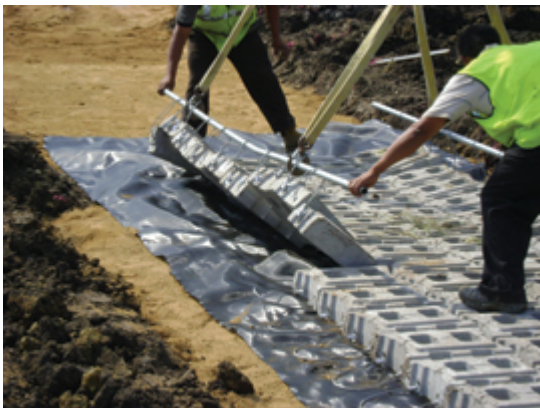
Photos: Submar One advantage that articulated blocks have over concrete is that the blocks move as the ground shifts and settles.
