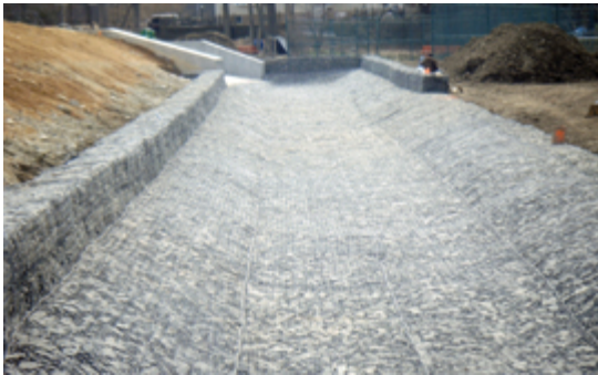
Photos: Maccaferri Gabions can be used to form natural drainage systems, minimizing the buildup of hydrostatic pressure on streambanks.
